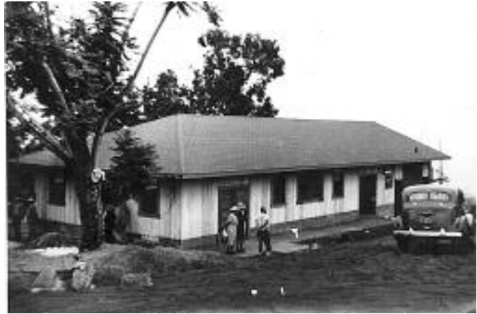
Construction of the Parish Hall.
